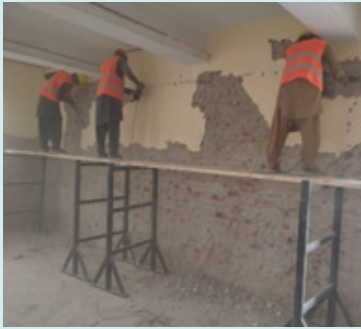
Fig-53a: Stripping wall plaster
