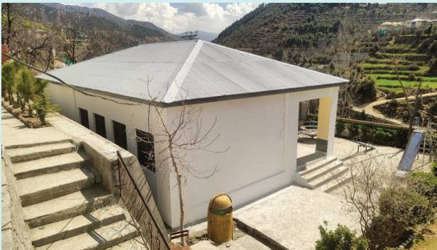
Fig-2c: Stone masonry building with light metal roof
