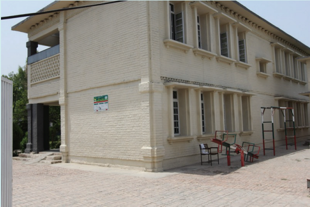
Fig-2b: Two-storey high brick masonry building
