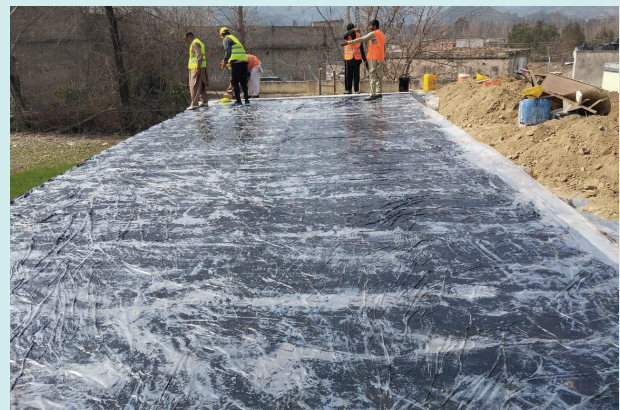
Fig-25: Roof treatment .
