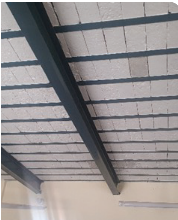
Fig-3: Iron Girder and T-iron roof
