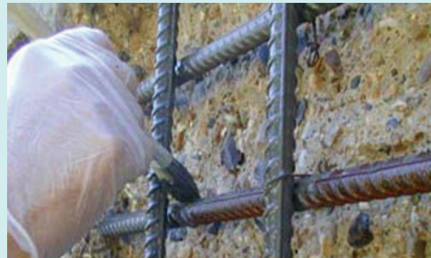
Repairing spalled concrete
