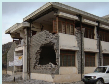
e. Topping of face-loaded wall
