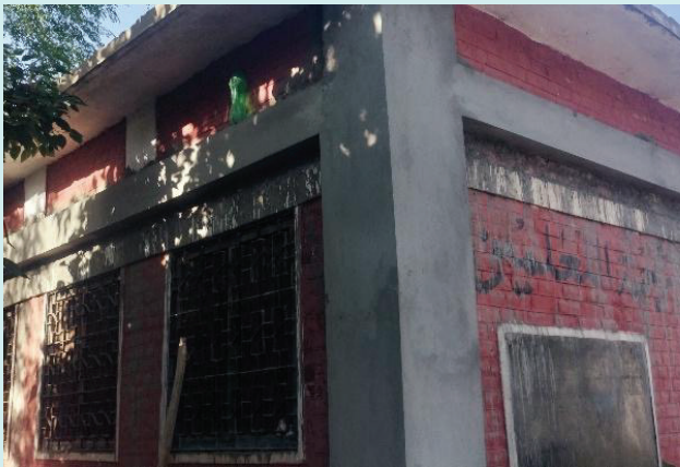
Fig-4a: A masonry building with seismic band at lintel level
