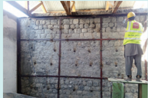
Fig-53f: Iron plates and wiremesh on stone masonry
