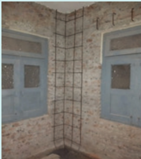
Fig-53d: Constructing splint :
