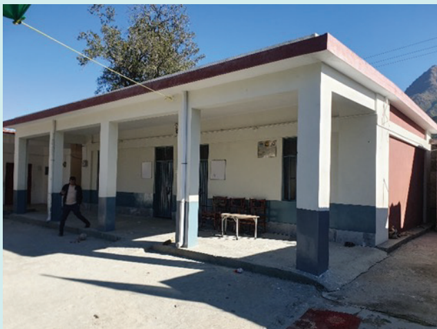
Fig-2d: A brick masonry building with RC slab roof
