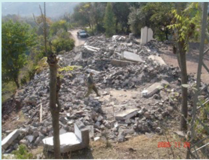
a. Destruction of school building during the Kashmir earthquake
