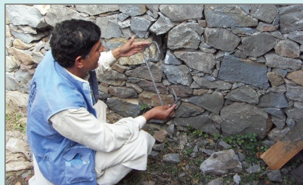
Fig-45: Installation of cross tie-Method-1
