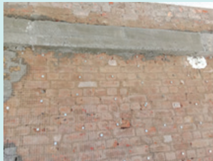
Fig-53e: Micro concreting bandage
