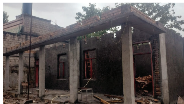
Fig-37a: A T-iron roof is being replaced with RCC slab
