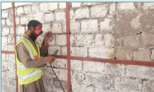
Fig-47: welding with iron flat with cross ties (method 2)
