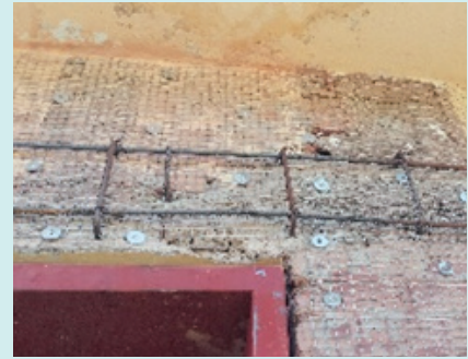
Fig-53c: Installing bandage bars
