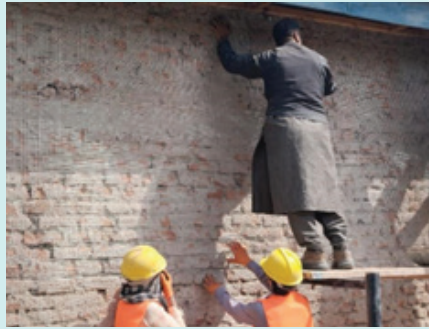
Fig-53b: Removing loose materials
