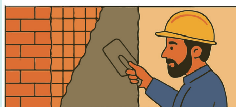
Apply First Coat Of Plaster
