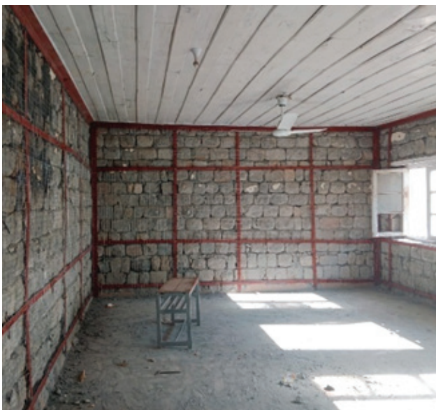
Fig-51: Steel flat retrofitting system under implementation
