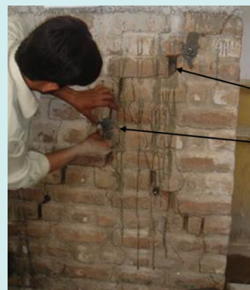
Fig-22b: Inserting and fixing the nozzles
