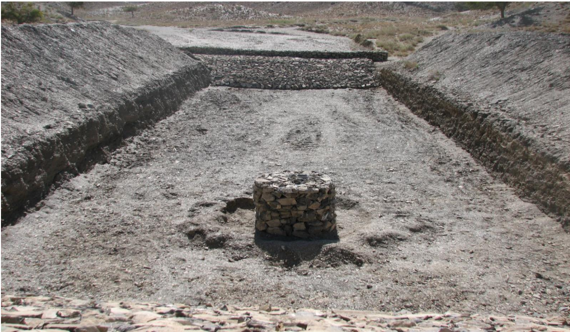
Figure 11: Inverted Well with Gabion/Check Structure
