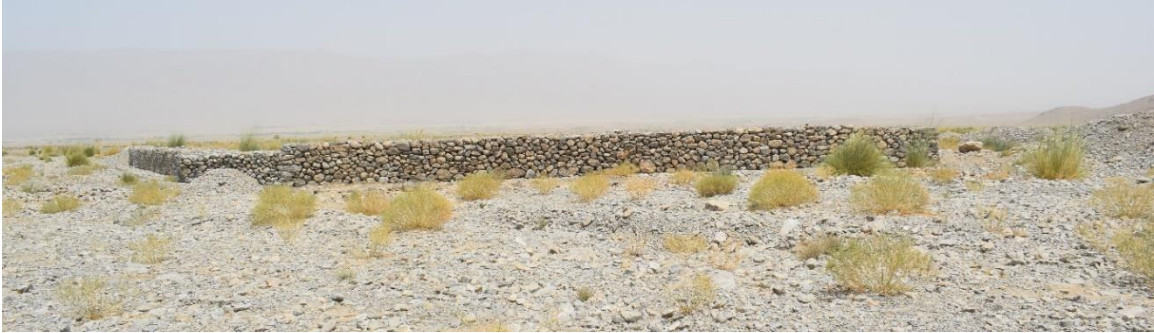
Figure 10: Gabion/Check Structure to Reduce the Speed of Flash Flooding
