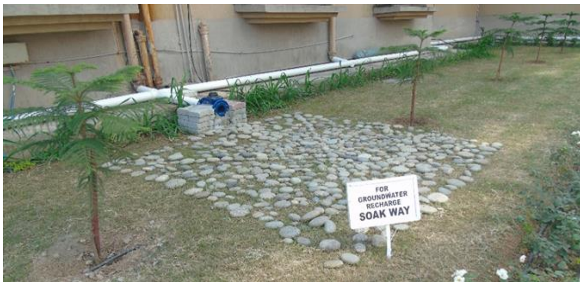
Figure 6: A surface View of Soak Way Pit
