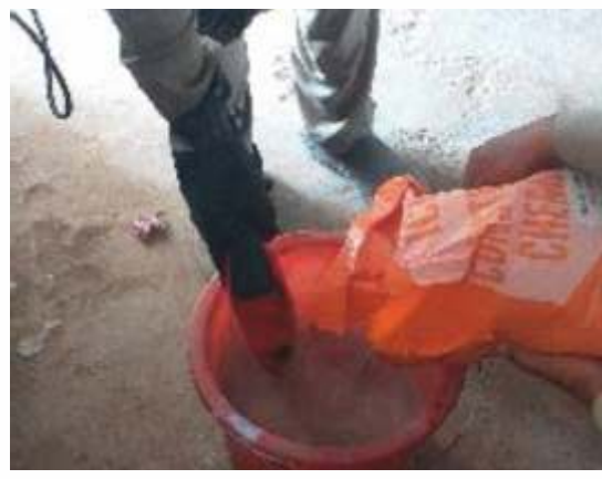
Mixing of waterproofing chemical (Liquid + Powder) application Through mechanical process
