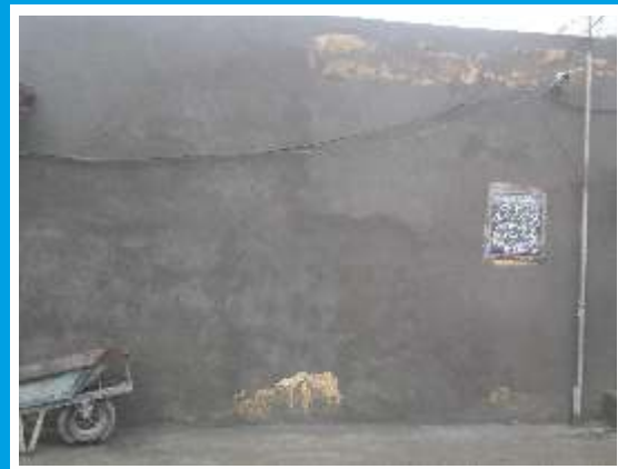
Fill voids with epoxy and apply fresh 1:3 c/s
