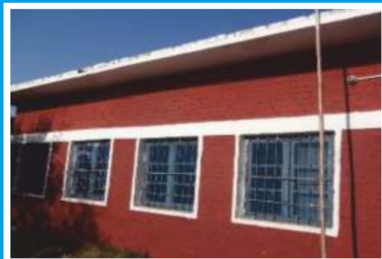
After Retrofit Works
