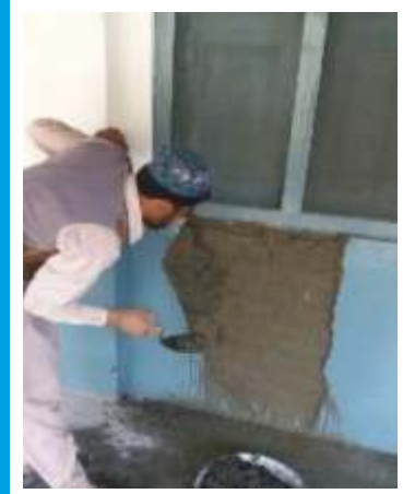
Chiseling of crack widely fixing of mesh for proper bonding Apply 1:3 c/s mortar of mortar
