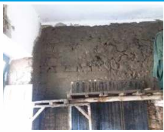
Dismantle existing loose plaster and fill epoxy on gaps/voids
