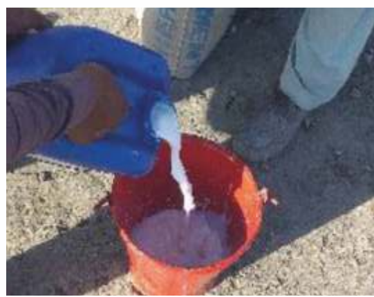
Prepare SBR mixing with cement
