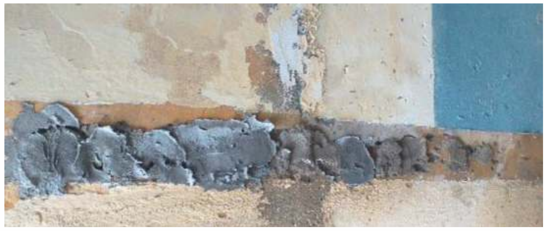
Filling epoxy on deep crack
