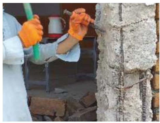
Eradicate existing buckle column excluding steel
