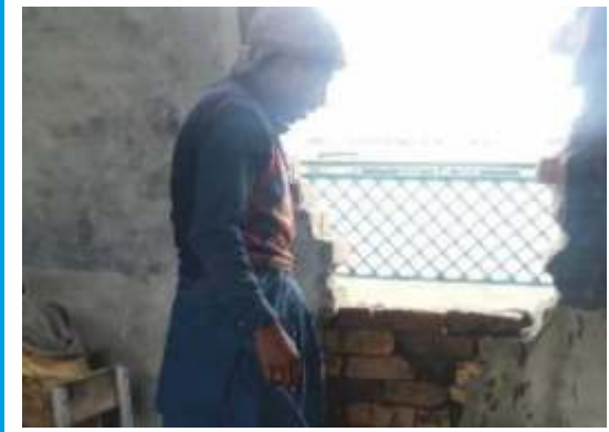
Opening of deep cracks for proper apply fresh prick masonry using bonding 1:3 c/s mortar
