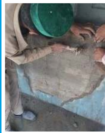
Chiseling of crack widely fixing of mesh for proper bonding Apply 1:3 c/s mortar of mortar
