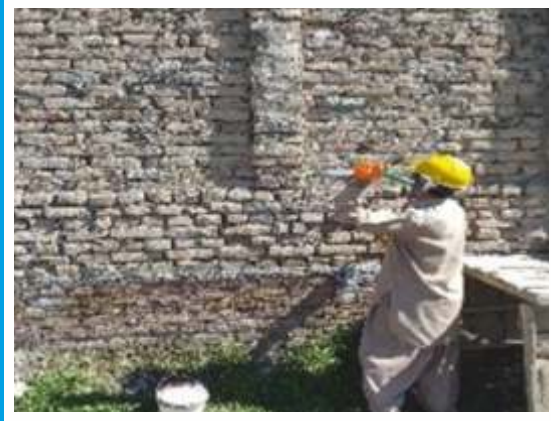
Demolish existing walls
