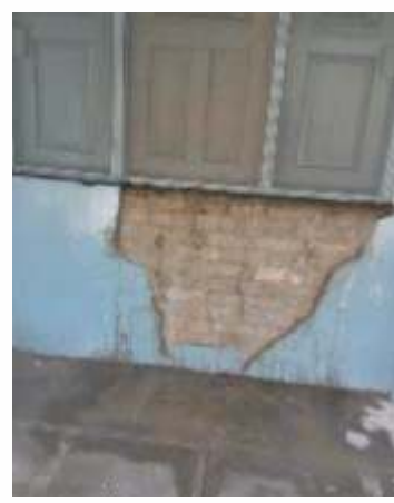
Chiseling of crack widely fixing of mesh for proper bonding Apply 1:3 c/s mortar of mortar
