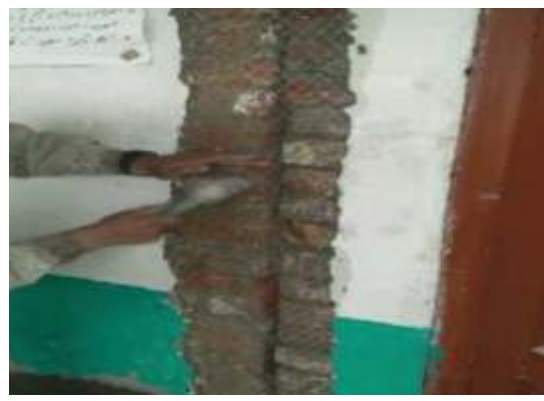
Fixing of mesh on joint
