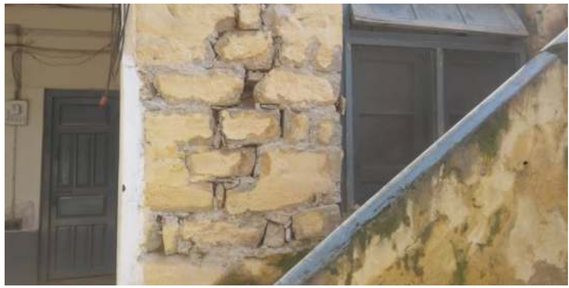
Removal of loose stones and fill mortar along with epoxy
