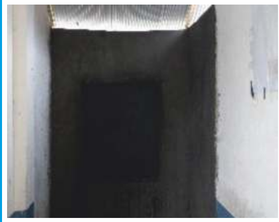
Covered with CGI shed and repair
