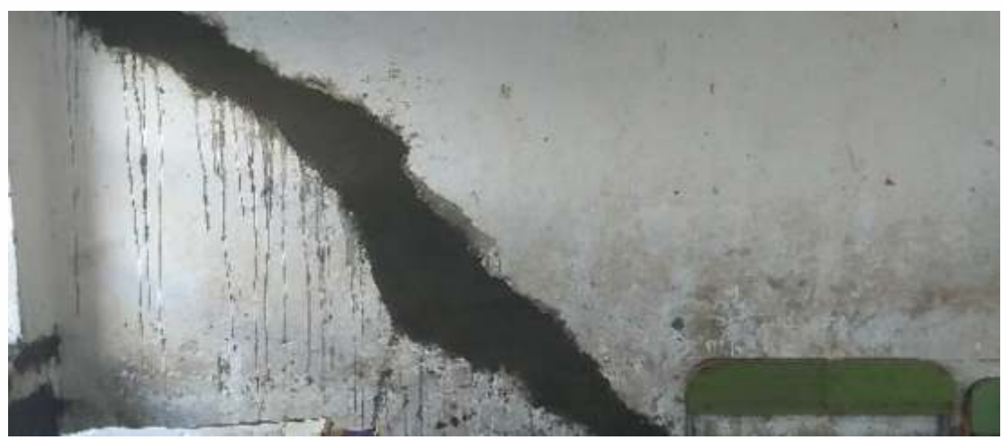
Retrofit of deep crack by filling epoxy and mortar
