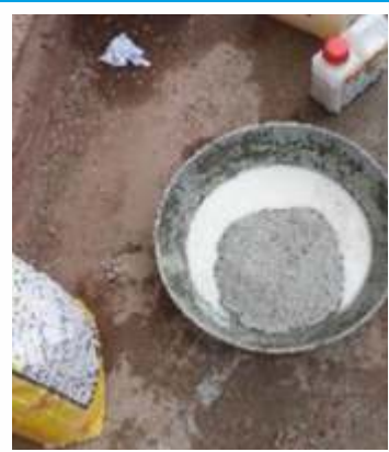
Prepare chemical combination of crush Anti-corrosion (liquid) and binding Agent (powder)
