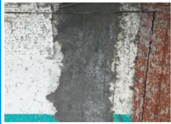
Apply mortar over bonding agent
