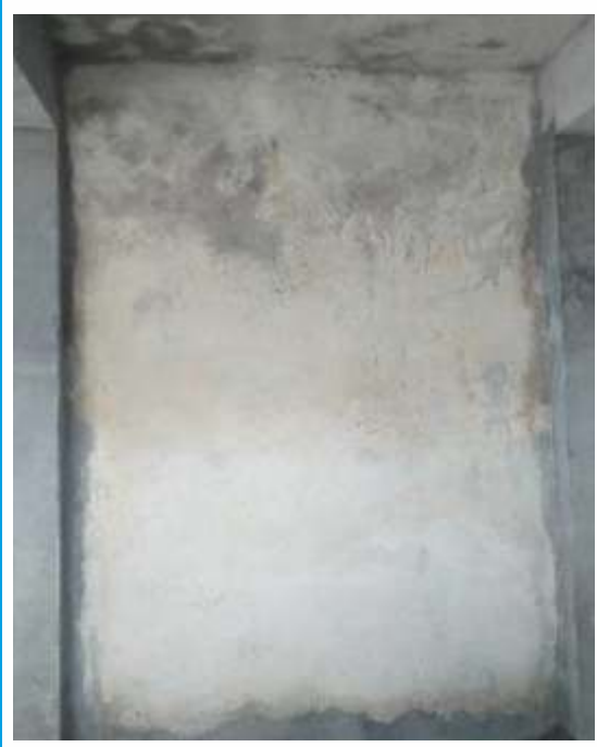
Apply white cement to strengthen plaster and avoid gradual erosion
