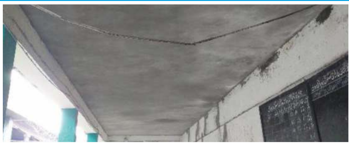
Retrofitting of ceiling through chemical process
