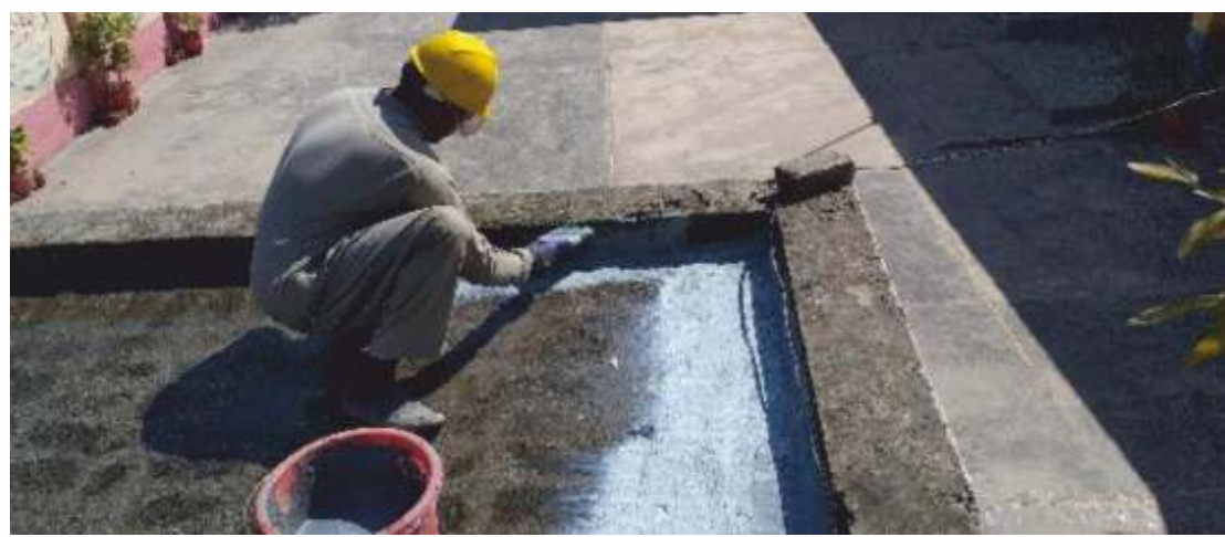
Apply two coats of water shield and allow drying
