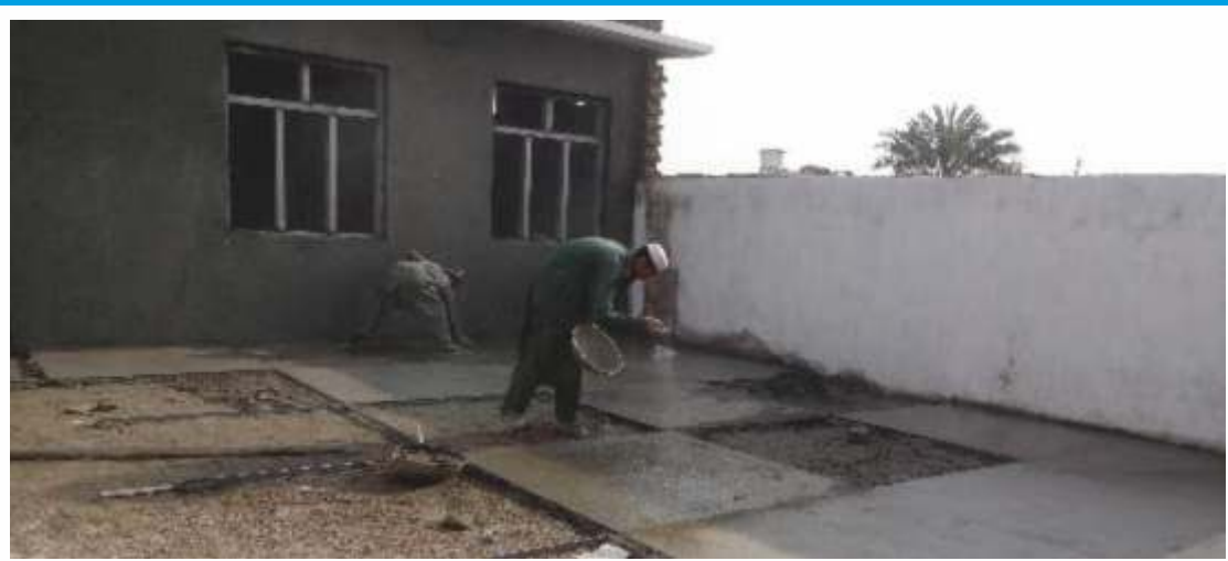
2" thick 1:2:4 PCC flooring in 5'x5' boxes using marble strips
