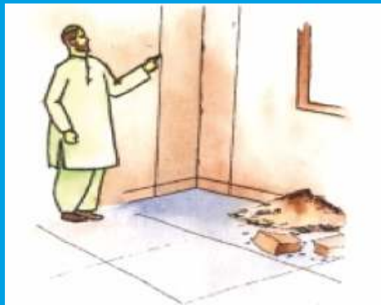
Marking boundaries of vertical rod concreting
