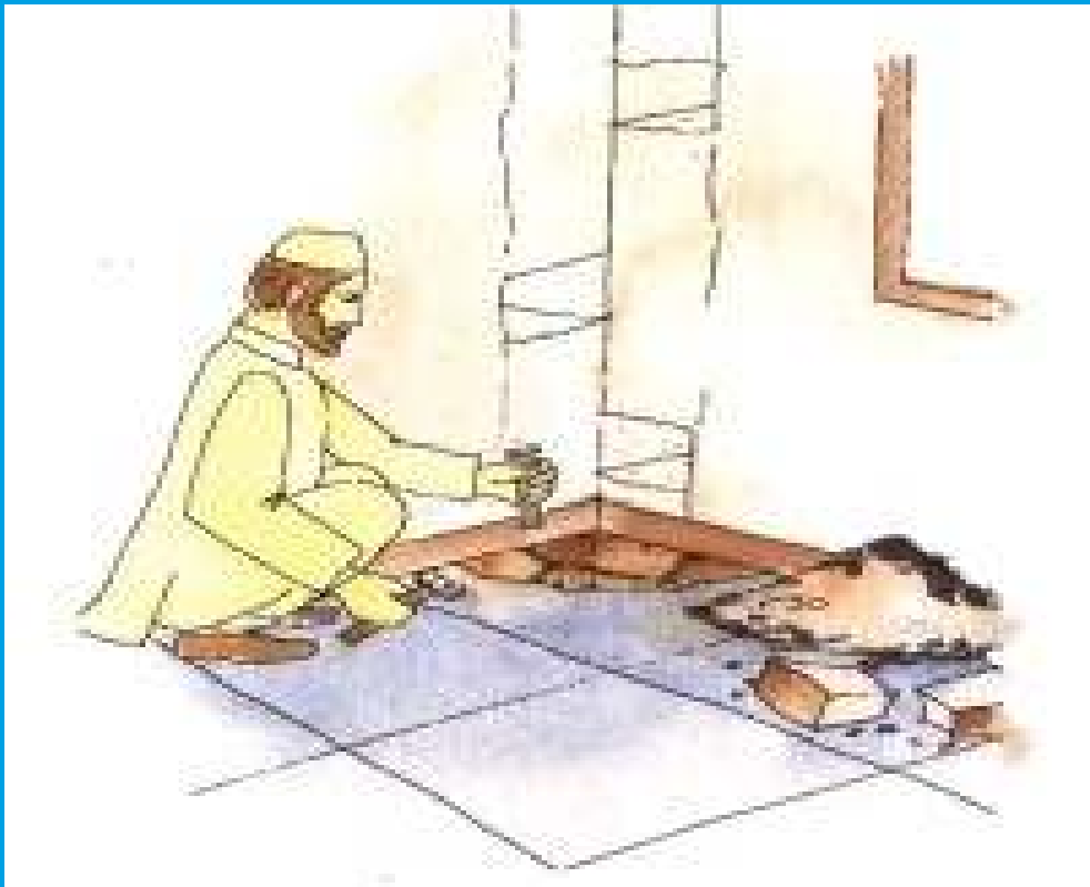
Breaking flooring and digging hole for vertical bar
