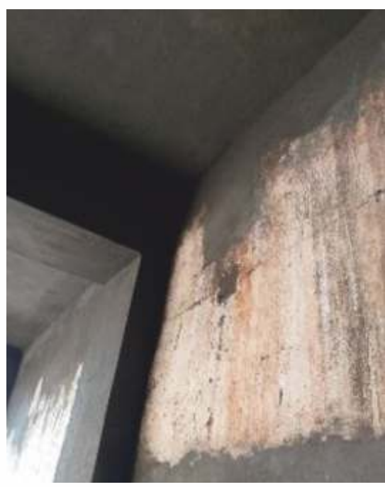
Apply anti corrosive agent and then apply mortar
