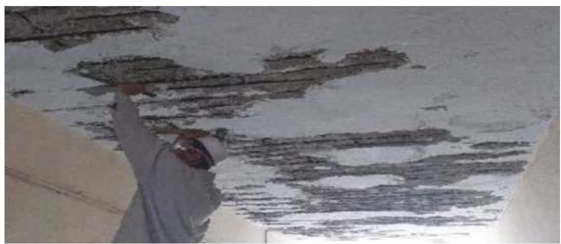
Chiseling of hollow plaster
