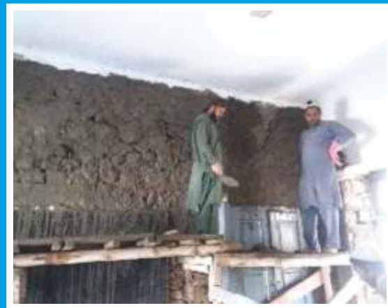
Dismantle existing loose plaster and fill epoxy on gaps/voids
