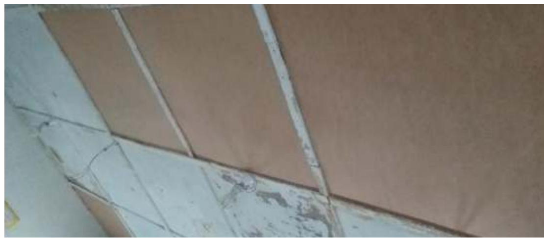
Replacement of damaged false ceiling
