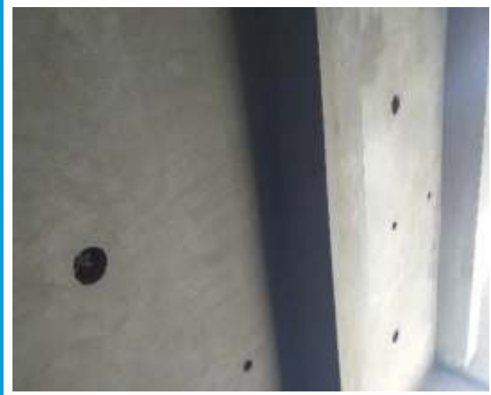
Apply SBR and then plaster using 1:3 c/s
