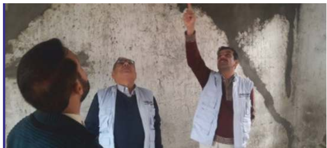
Retrofitting of cracks by filling epoxy and mortar; Repairing of windows
