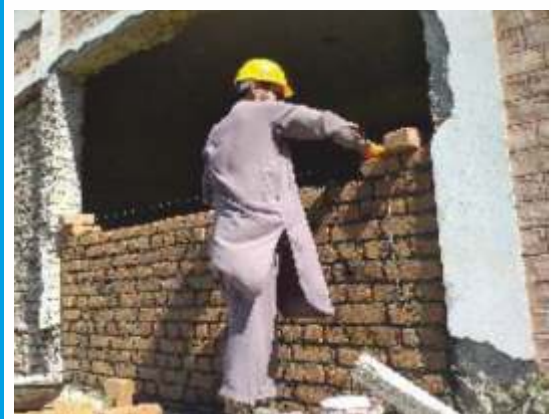
Provide fresh masonry using 1:3 c/s
