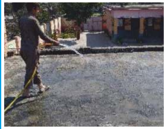
Curing of slab prior to water shield
