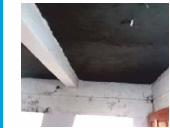
Apply SBR and then 1:3 c/s mortar
