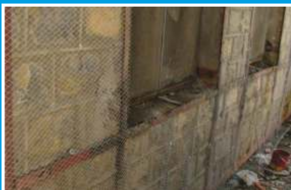
Installation of vertical and horizontal metal strips
