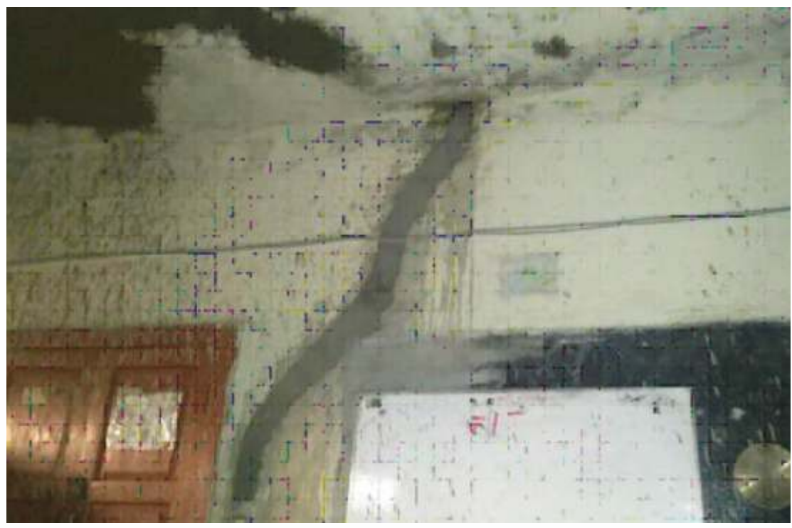
Cracks retrofitted by filling epoxy
