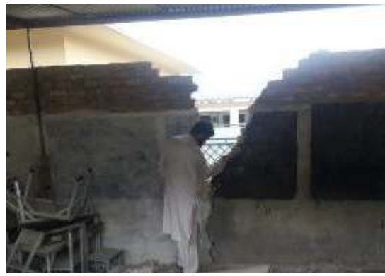
Opening of deep cracks for proper apply fresh prick masonry using bonding 1:3 c/s mortar
