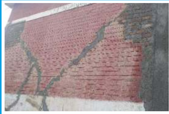
After Retrofit Works
