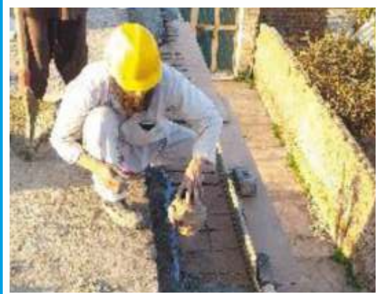
Retrofitting of RCC projections using SBR and concrete
