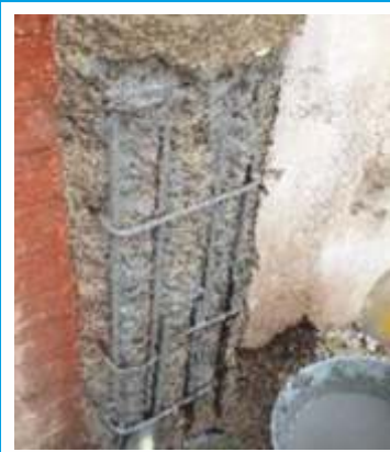
Apply chemical over column
