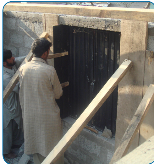
5- Fix shuttering on both side of wall. On one side the shuttering plank should cover the complete height of the opening.
