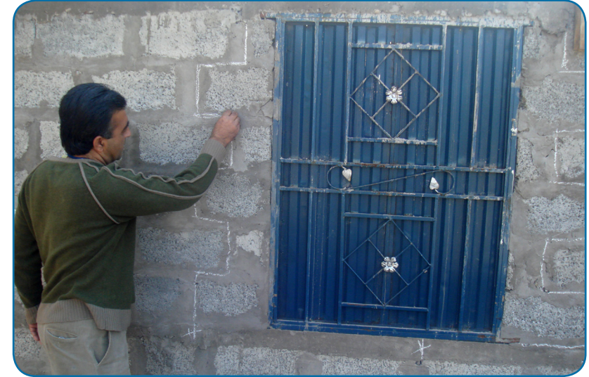
1- Mark the blocks on both sides which should be taken out in toothed pattern for providing reinforcement.
