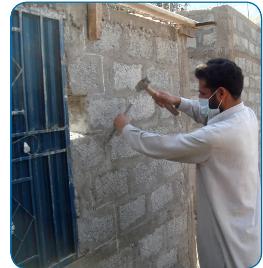
2- Take out the marked blocks with the help of chisel and hammer. (If the window or door frame is not fixed than support the lintel firsts)
