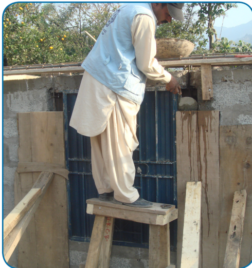
6- On the other side of the wall the shuttering should be fixed with an opening on the top for pouring concrete.
