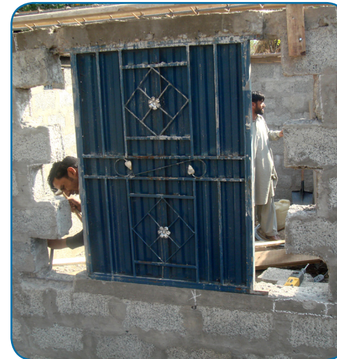
3- Chisel the sill band on both sides upto 2 ft to embed the vertical reinforcement in the sill band.
