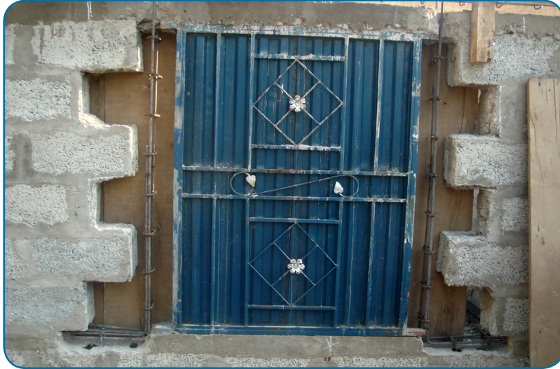
4- Place 2-#4 main bars with #2 @6" spacing stirrups.
